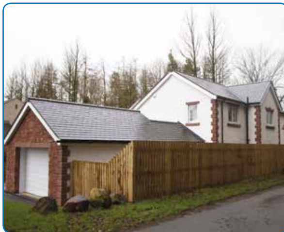
The complete America Field project, a modern, attractive 3 bedroom property.
